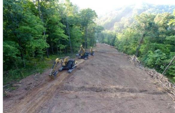
Engineered access roads with water diversions and soil controls
